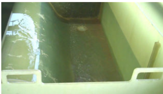
Figure 8: Organic overflow weir, showing smooth flow and no air entrainment
