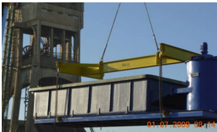
Vacuum infusion of the resin results in a fully competent, strong, smooth-surfaced product with no air voids anywhere in the construction. The final completed settler was attached to the pumper-mixer tank, secured to its base frame and moved into position as one unit, shown in Figure 10.
