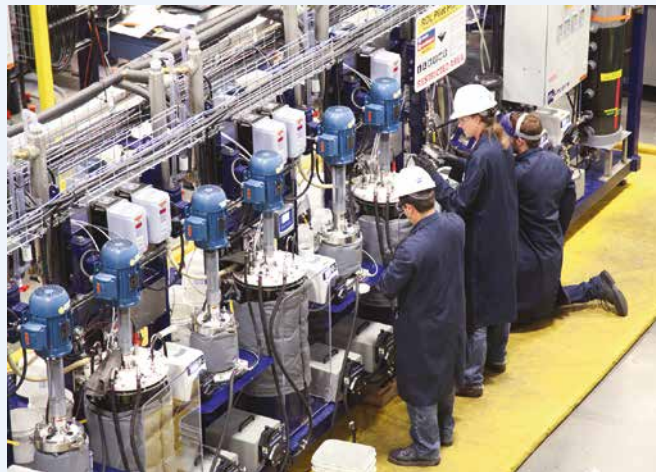
ROL pilot plant being installed in Utah, USA. Photo: FLSmidth
